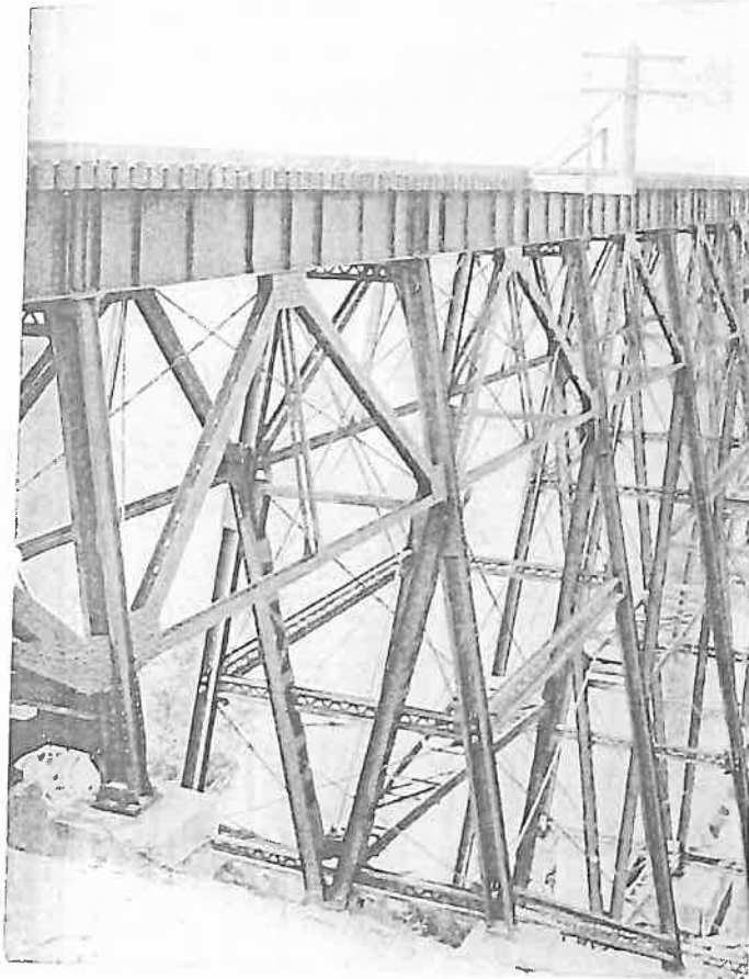
Details of Reinforced Viaduct, Pere Marquette.
